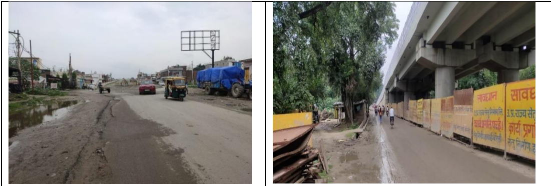
Figure 2: Flyover construction at Lal Phatak Railway Crossing
