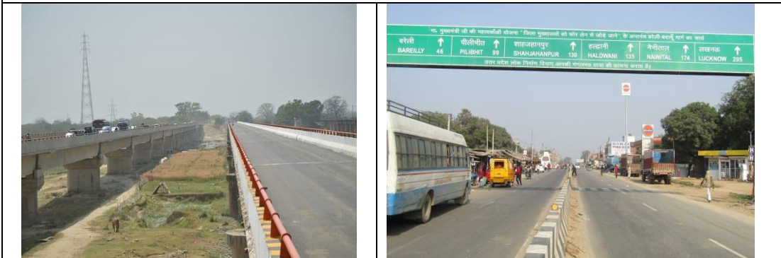
Figure 3: Major Bridge along Ramganga River
